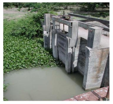
Figure 1. Head gate inlet into canal B (one operational gate).
