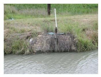
Figure 10. Root-gate usually made of wood.
