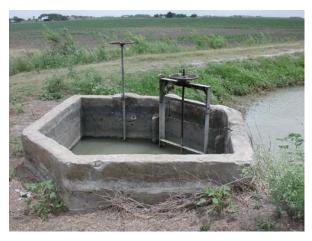
Figure 9. A box head gate situation that typical occurs at the beginning of a canal or after a road crossing. This controls downstream, levels and supplies usually two farm turnouts.
