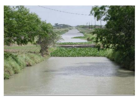
Figure 2. Culvert clogged by aquatic vegetation (Water Hyacinth)
