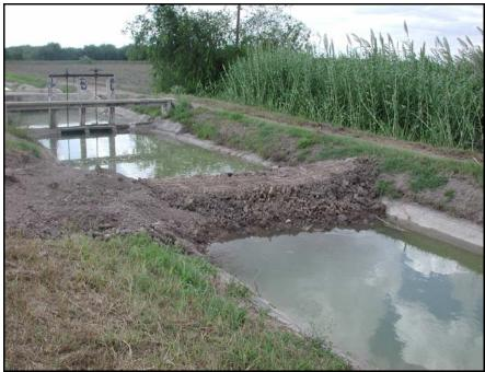
Figure 1. Earthen dam constructed on lateral A - Stewart Rd.
