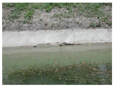
Figure 5. Large crack in the canal lining and aquatic vegetation growing from the bottom of the canal (lateral A - Stewart Rd)
