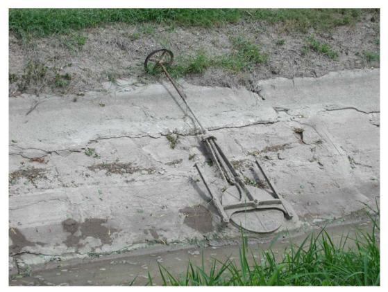
Figure 9. Cracking of lateral A - Stewart just down stream of the test section.
