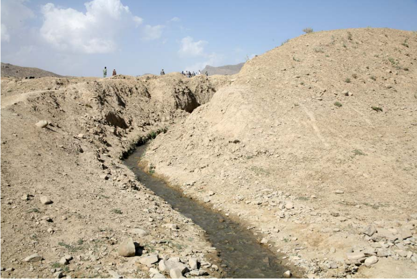
Photograph 2. Trench that carries the water from the NW Karez down slope to the village.
