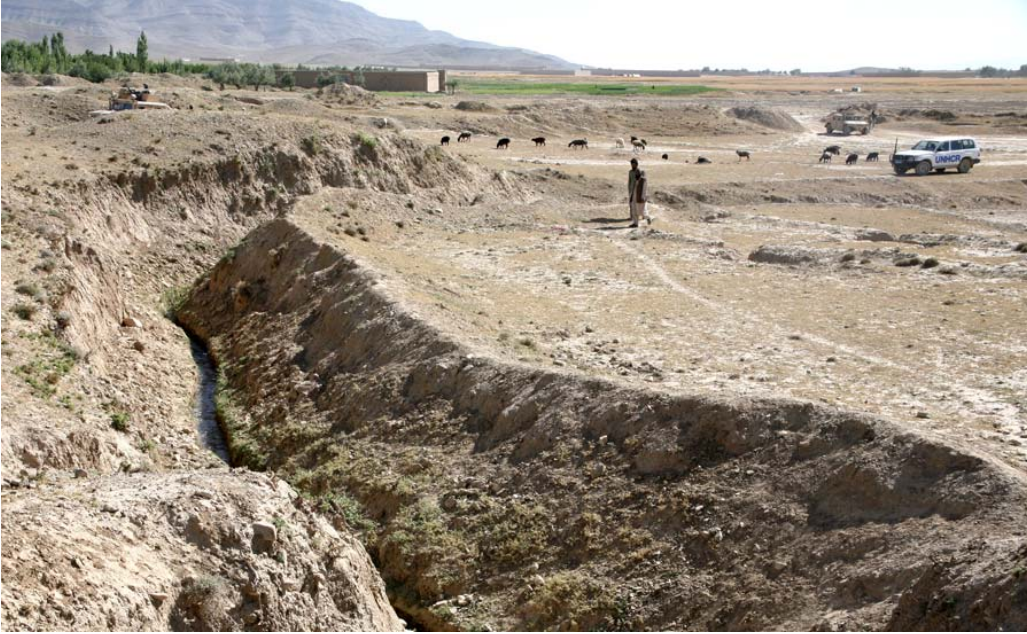
Photo. 4. The trench of the NW Karez. In the distance, (beyond the UN vehicle) the humvee is parked near the outlet for the HLZ Karez. To the left of the humvee is the line of access shafts marking the path of the HLZ Karez leading to the helicopter landing zone of the Gardez FOB.
