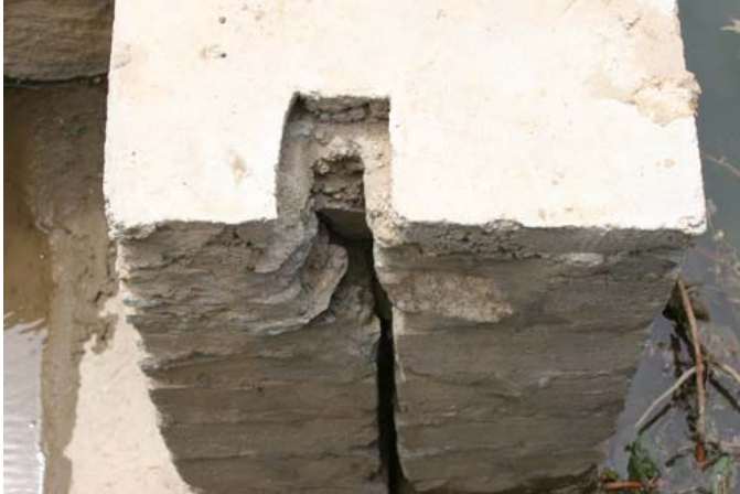
Non-vertical groove, impossible to insert gate
