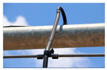
Figure 9. Truss rod hose clamps/slings.
