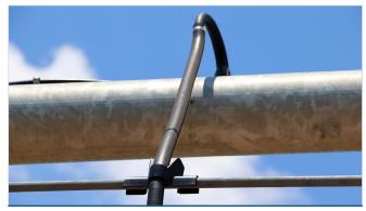
Figure 9. Truss rod hose clamps/slings.
